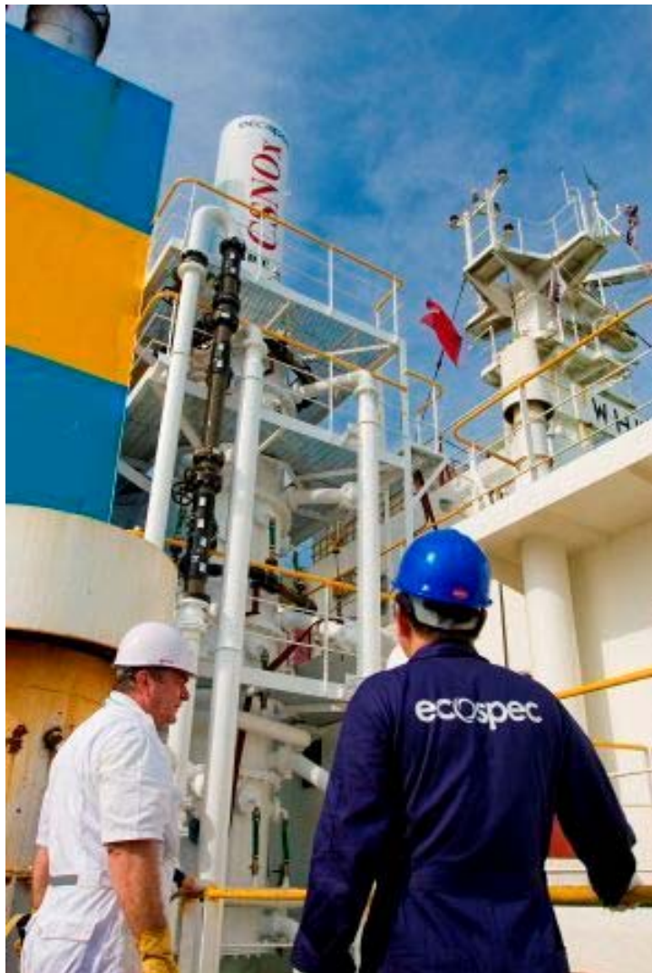
Caption: CSNOx onboard 100,000-tonne Aframax tanker for first load point verifications
