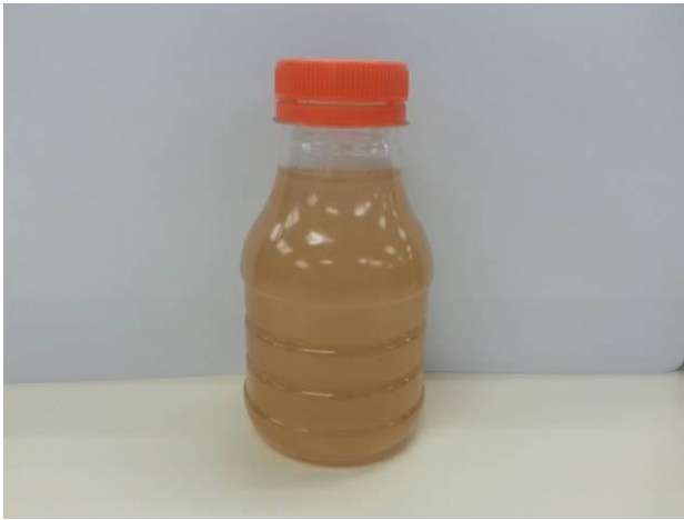
Boiler water before ScaMag treatment (May 2015)
